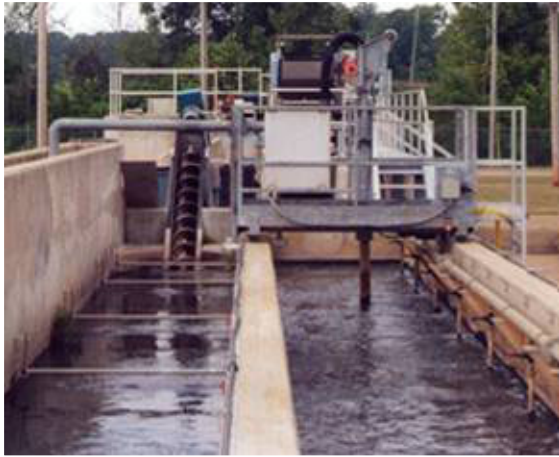
Figure 7 – Typical Traveling Bridge Grit Removal System Installation (Schreiber, Inc.)
