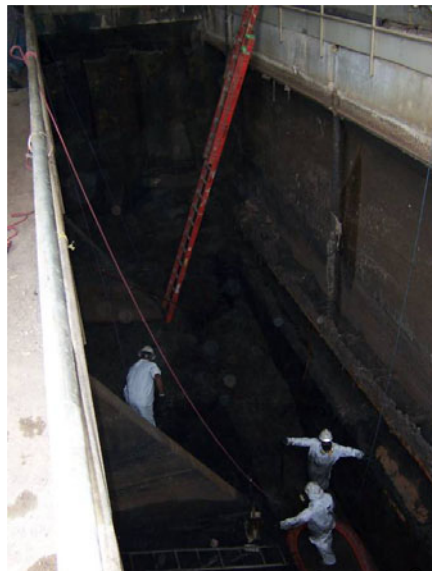
Figure 3 - Manual Grit Removal in Grit Chamber Building No. 2
