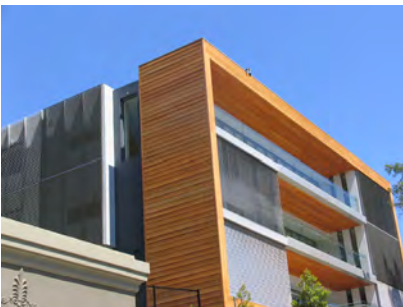
Deep ledges protect glazing from energy loss and gain
