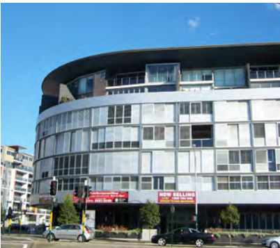
Development on a busy road is articulated using recessed balconies, operable louvres and a roof overhang
