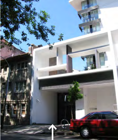
The vehicular entry is treated as part of the elevation. It narrows the width of the entry and defines an opening in proportion to the other facade elements.
