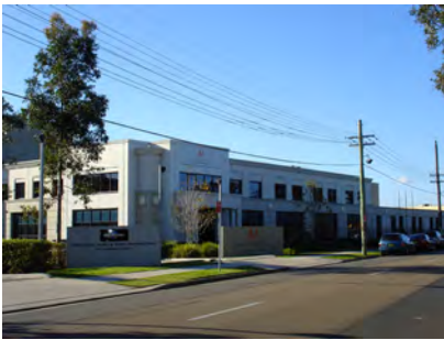
Industrial development includes building articulation and landscaping
