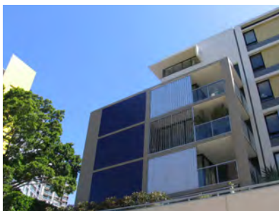
Operable louvres provide climate control
