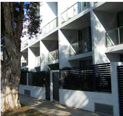
Ground floor apartments have direct access to the street
