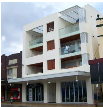
Building articulation in a heavily modelled street wall building
