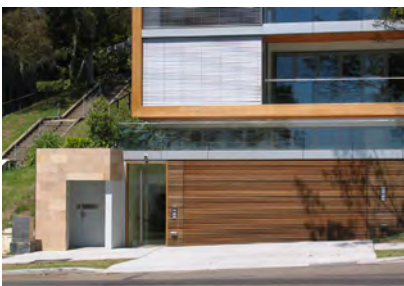
The use of sandstone at ground level provides a solid building base and enriches the public domain
