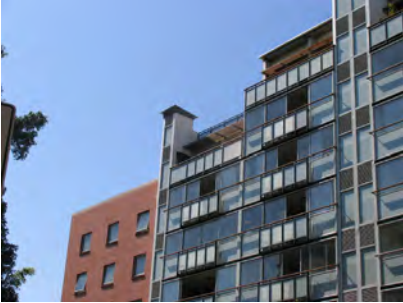
Loggias provide protection from road noise
