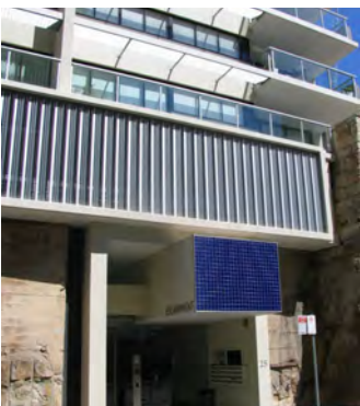
Building entries are clearly defined
