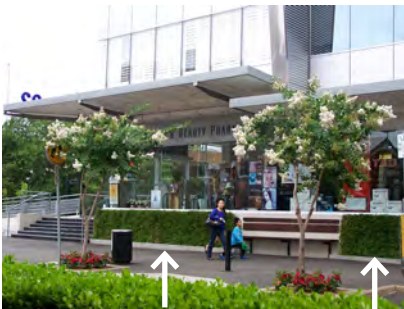
Planting screens above ground basement car parking walls
