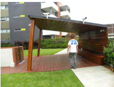
High quality usable communal open space provides recreational opportunities and enhances the built environment and residential amenity
