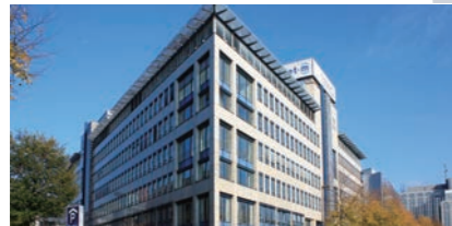
R&D Center in Fujitsu General (EURO) GmbH (Germany)
