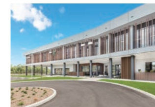
Fujitsu General (Aust.) Pty Ltd. (Australia)
