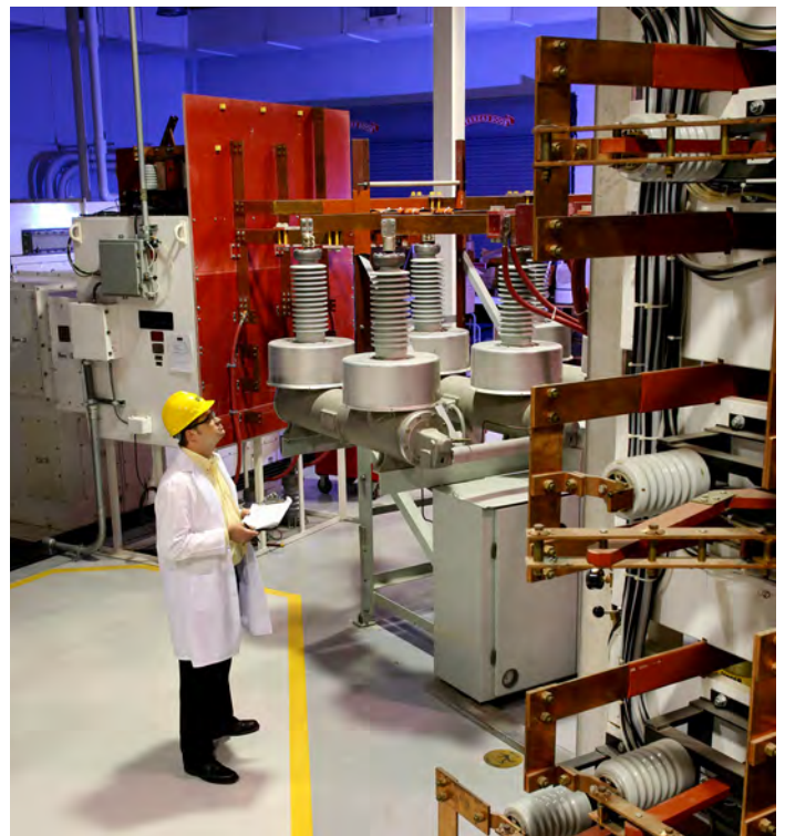
The Eaton Bussmann Division’s Paul P. Gubany Center for High Power Technology is the electrical industry’s most comprehensive facility for testing and certifying device and equipment SCCRs. Capable of performing electrical tests up to 600 V three-phase, 300 kA of short-circuit current for meeting ANCE, ANSI, CE, CSA, ETL, IEC and UL testing requirements.
