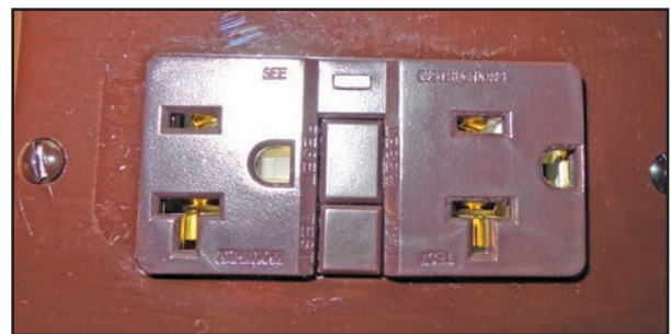
Figure 9-13: GFCI receptacle
