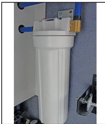
Figure 13-7: Water filter
