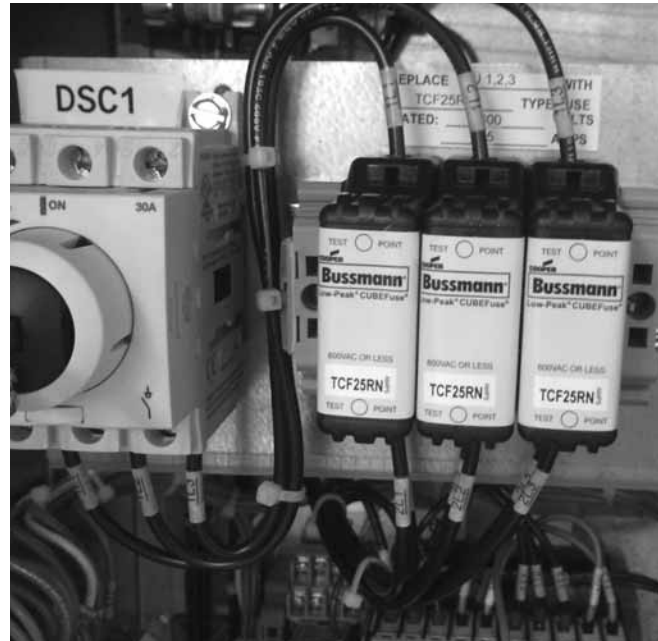
Figure 9. Fused disconnect
