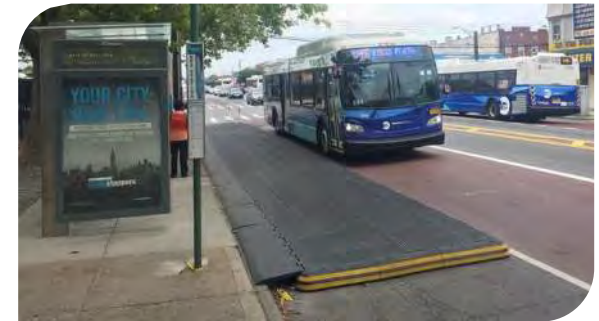
Above Top: The City of Fremont has used a combination of painted bulb outs with self-watering landscape planters to achieve this effect. Above: Prefabricated boarding islands or parklet-style boarding islands can be used to extend the sidewalk and allow buses to stop in line to improve transit reliability. Photo credit: www.zicla.com
