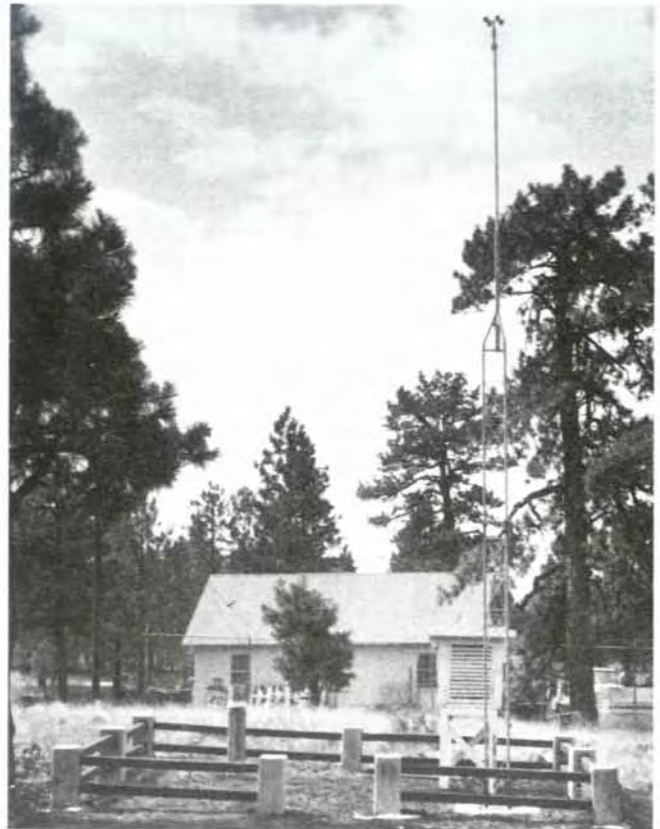
Figure 17.2(A and B) —Anemometer installations with height adjusted upward because of nearby trees.
