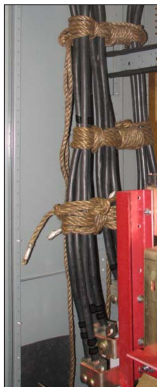
Figure 25 – Cable Restraint Example
