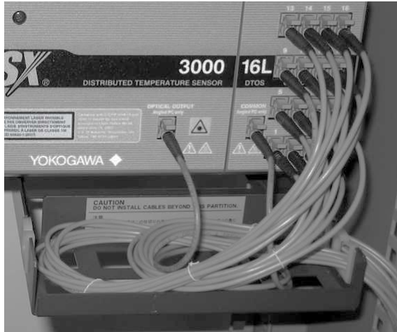
Figure Example of Cable Routing using the DTRK10
