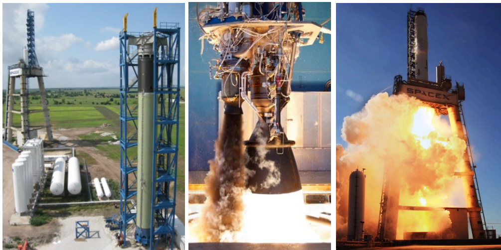
Figure 6-10: SpaceX Texas test facility and test operations
