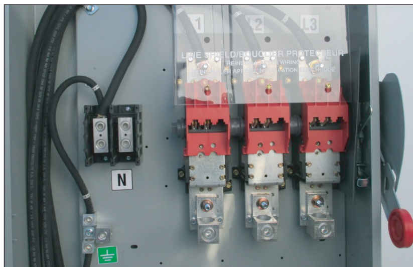
Figure 21 - Generator Output Connection Lugs
