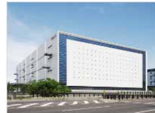
New building at SEND's Motomiya site
