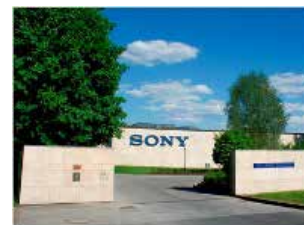
Sony DADC's site in Anif, Austria, one of the sites in Europe that uses 100% renewable energy
