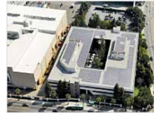
Solar power generation facility installed on the roof of SPE's headquarters
