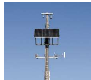
Coastal tsunami monitoring system in Higashi Matsushima City in Miyagi Prefecture
