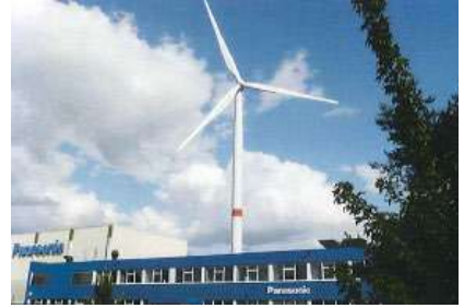
Wind power generation system in PECBE
