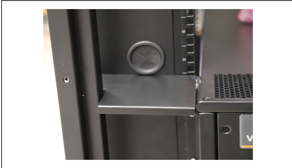
Figure 4.3 Air Baffle Installed—800 mm (31.5 in.) Rack
