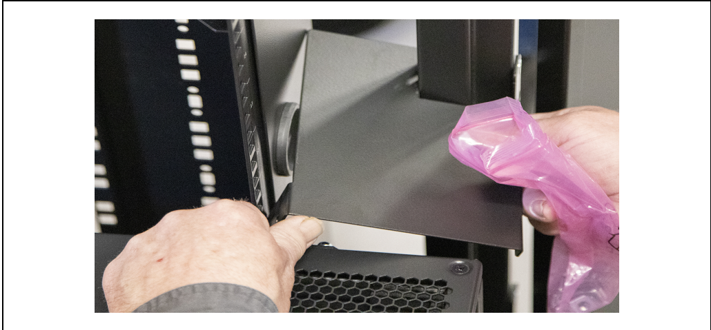
Figure 4.2 Attach Air Baffles—800 mm (31.5 in.) Rack
