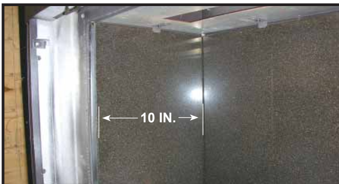
Figure 8. View of Back and Side Piece Installed.
