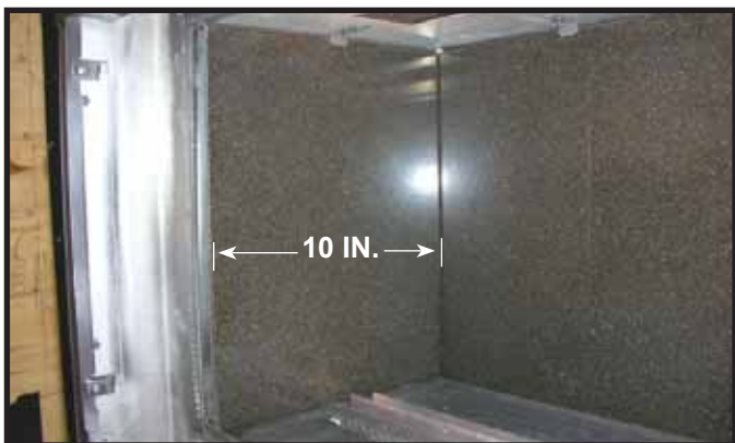
Figure 13. View of Back and Side Pieces Installed.
