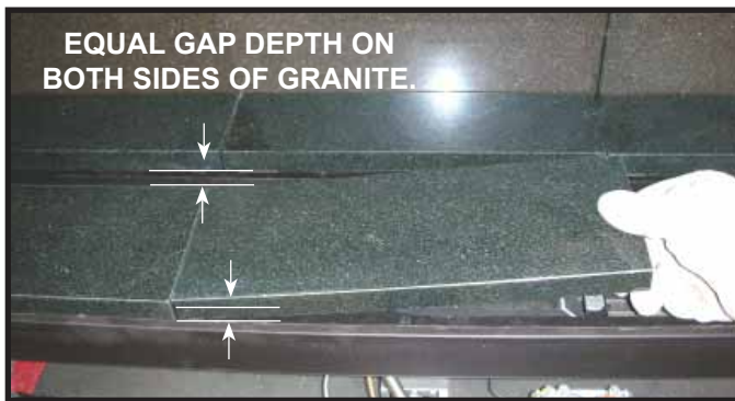
Figure 16. Installing Inner Front Granite Pieces.
