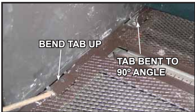
Figure 7. Bend Tabs Up to a 90 Degree Angle.
