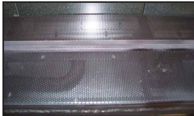
Figure 15. Base Mesh Installed.
