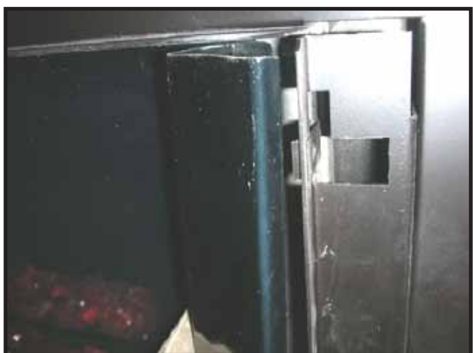
Figure 9. Installing Outside Corner Trim Piece onto Clip.
