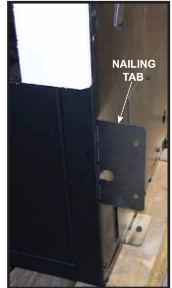
Figure 6.4 Nailing Tabs Installation Position
