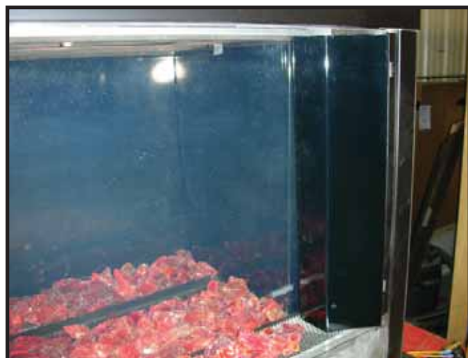
Figure 10. Outside Corner Trim Piece Installed.
