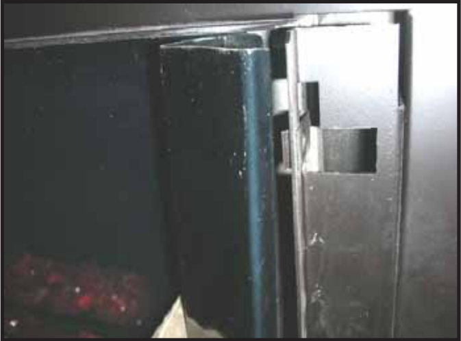
Figure 16. Installing Outside Corner Trim Piece onto Clip.
