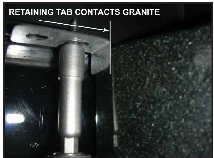
Figure 21. Placing Outer Corner Granite Trim Piece.
