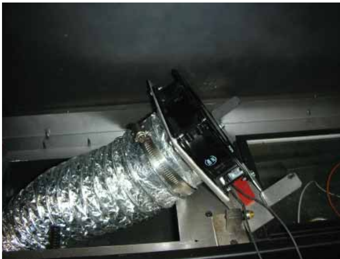
Figure 8.16 Blower Removal Through Hole in Firebox
