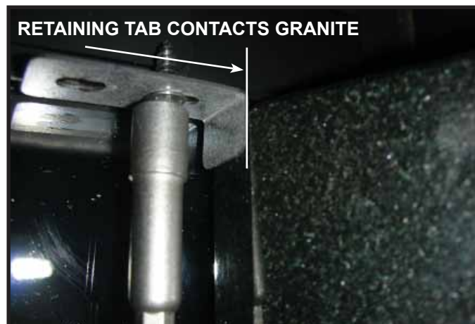
Figure 10. Placing Outer Corner Granite Trim Piece.
