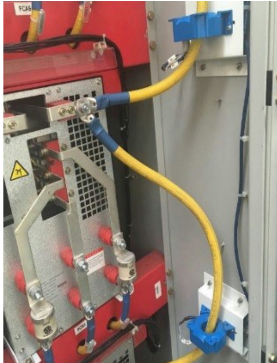
Figure 18 - Star Connection Cable (UL)
