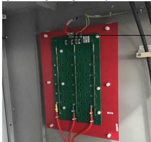
Figure 2 - Voltage Sensing Board Output Connection Cable (IEC)
