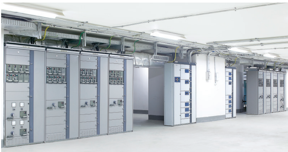
Figure 4-01 Example of switchgear room layout
