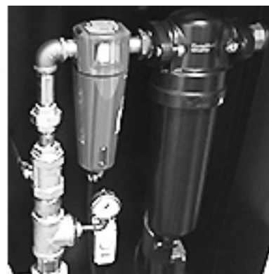
Figure 4-2. Coalescing Filter and DPI
