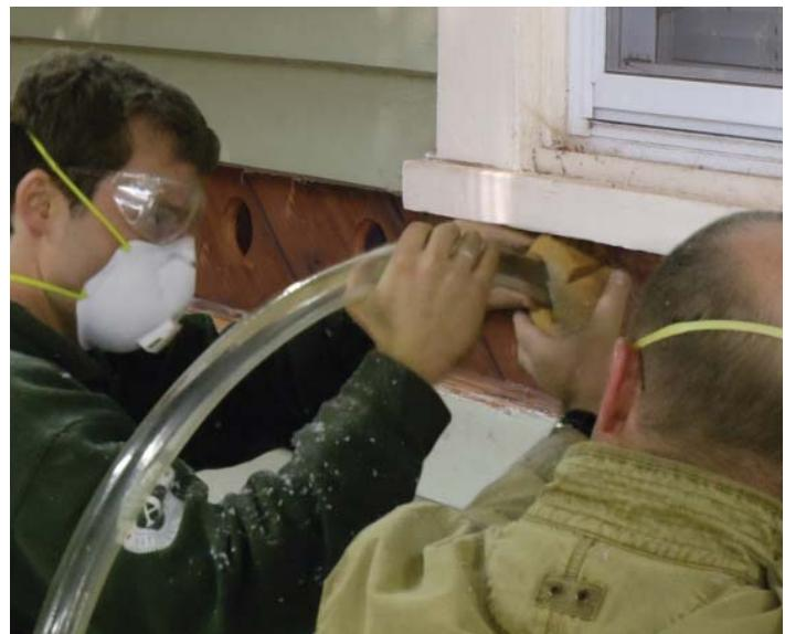
6. Insert cut end of the tube through the filter into the 2 1/2-inch drilled hole and feed to within 6-inches of the top of the stud cavity. Note any fire stops or other obstructions. Drill additional holes as needed if obstructions are present.
