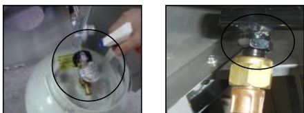
Gas Connection Leak Check
