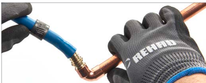
Fig. 4.12: Removing pipe from LF brass fitting
