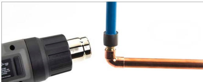
Fig. 4.11: Heating EVERLOC+ compression sleeve with heat gun
