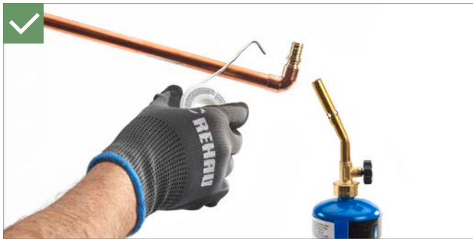
Fig. 6.19: Solder prior to making EVERLOC+ connection
