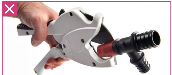
Fig. 4.10: DO NOT cut RAUPEX pipe from fitting
