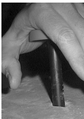
Figure 5.1 Pressing the sleeve into the hole
