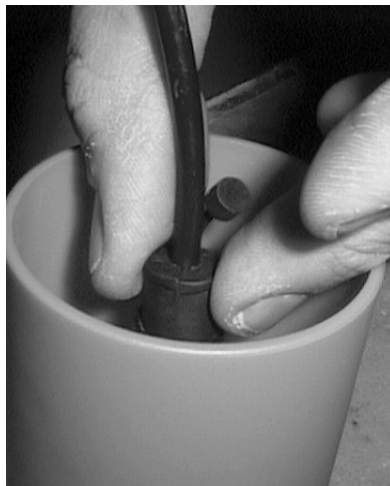
Figure 5.3 Sealing the sleeve with a plastic plug
