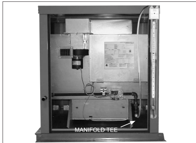
Figure 15.2 - Maxitrol Modulating Valve Adjustments
