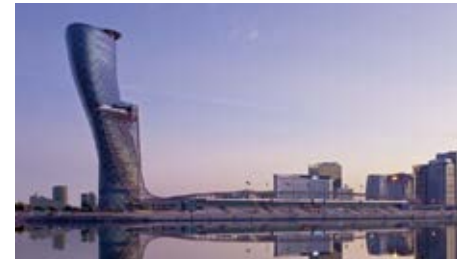
Hyatt Capital Gate Hotel, Abu Dhabi. Hansgrohe products: Raindance S 240 Air overhead shower. Photo: abudhabi.capitalgate.hyatt.com
