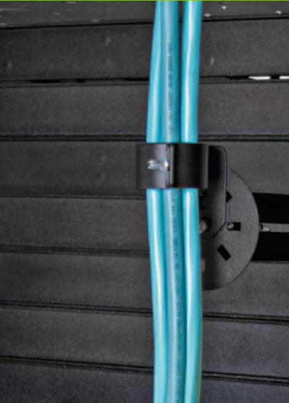
Rack-Mount Universal Clamp Kit Installed
