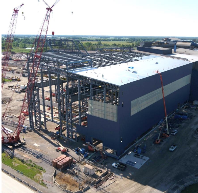
Melt shop building cladding underway
