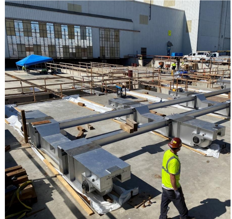
Installation of shuttle furnace underway
