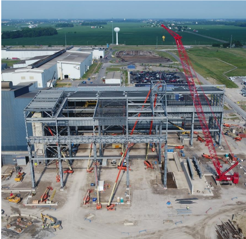
Melt shop building frame nearing completion
