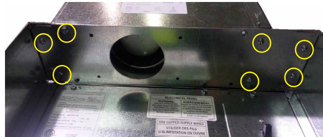
FIGURE 18 - DAMPER PLATE FASTENERS
