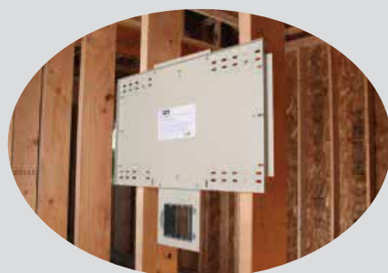
Fast and easy: The back plate installs directly to the framing studs during the rough-in construction phase.
