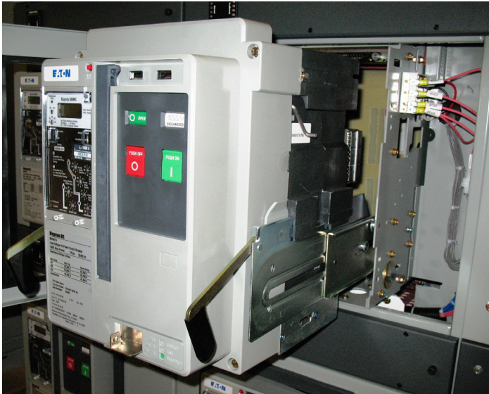
Figure 9. Magnum DS breaker on extension rails
