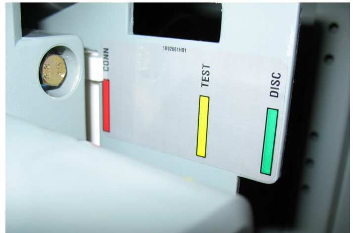
Figure 11. Magnum DS breaker position label
