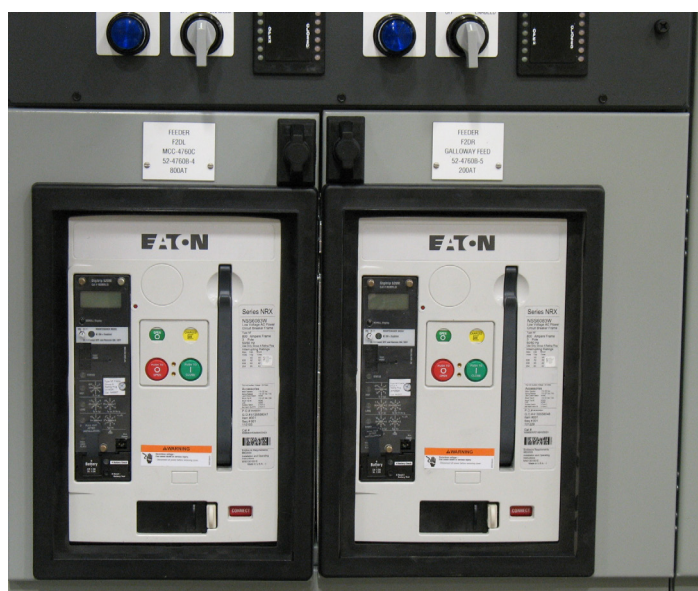
Figure 8. Series NRX breakers in connected position
