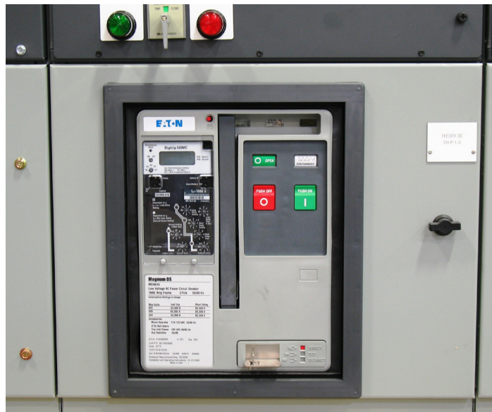
Figure 7. Magnum DS breaker in connected position
