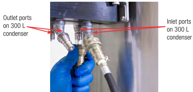
Figure 2.11. Attaching TCU lines to a condenser on a 300 L S.U.F. unit.
