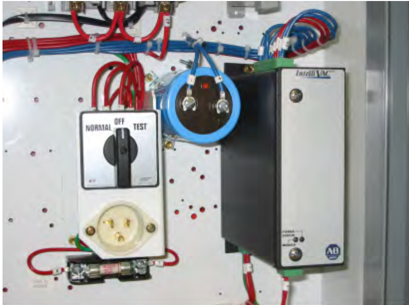
Figure 4 - Typical IntelliVAC Installation within a Bulletin 1500/1900 MV Controller (Shown with optional external capacitor)
