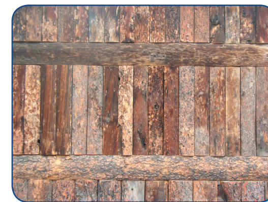
“Grand Lake wooden slab siding”
