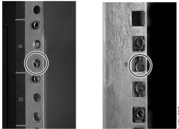
Figure 36. Incorrect connector locations
