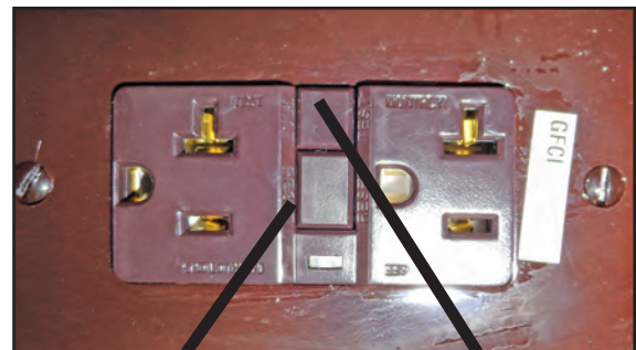
Figure 9-3: GFCI receptacle
