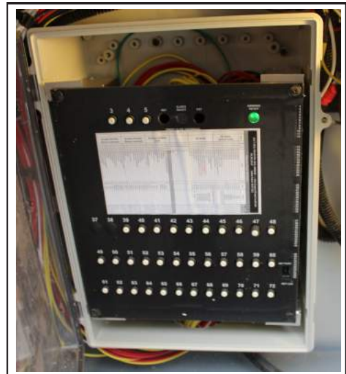
Figure 9-7: Circuit breakers
