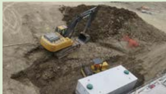
Preparing to install a rainwater recycling system
