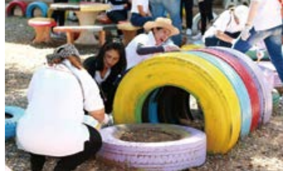
Maintenance and repair of school facilities by employees and neighboring residents landscape
