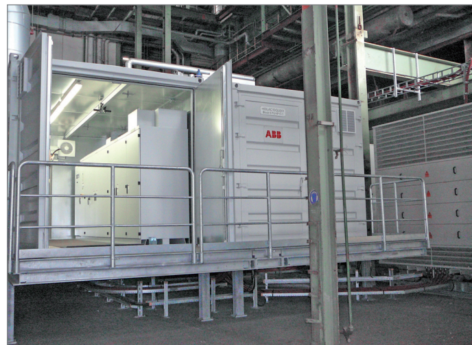
The water-cooled ACS 1000 medium voltage AC drives were installed ready for connection in special, fully air-conditioned containers
