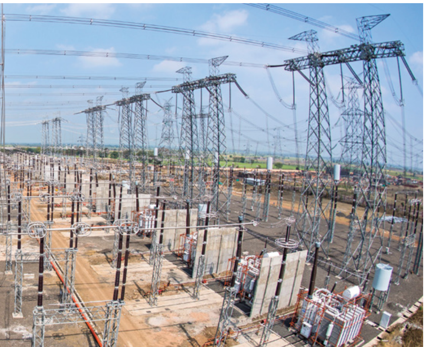
▲ Air Insulated substation at Bina
