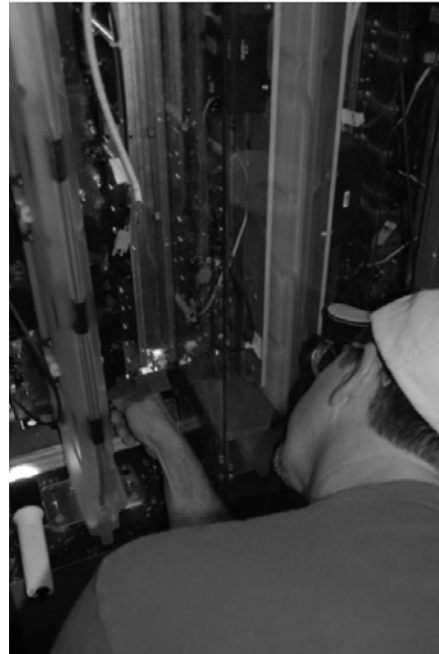
Figure 26. Remove bolts to capacitor
