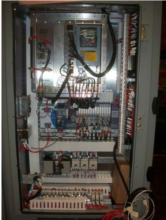
Figure 12. SC9000 EP AFD low-voltage door open
