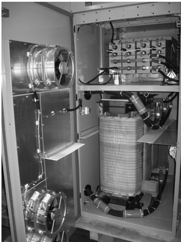
Figure 87. Sine filter with filter fans shown
