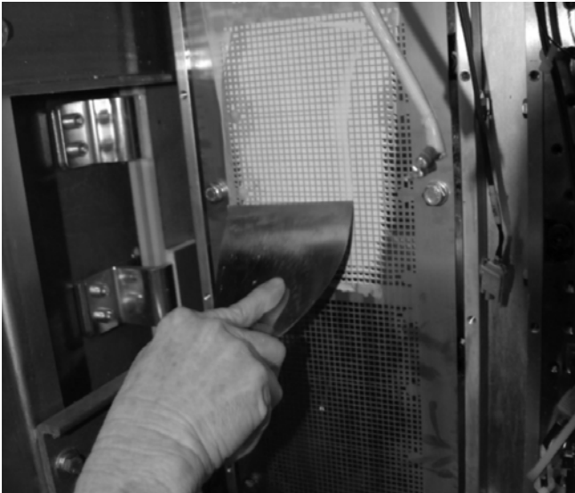
Figure 29. Apply thernal paste
