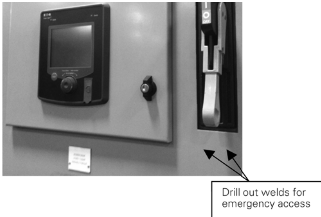
Figure 24. Drill location for emergency entrance to cabinet
