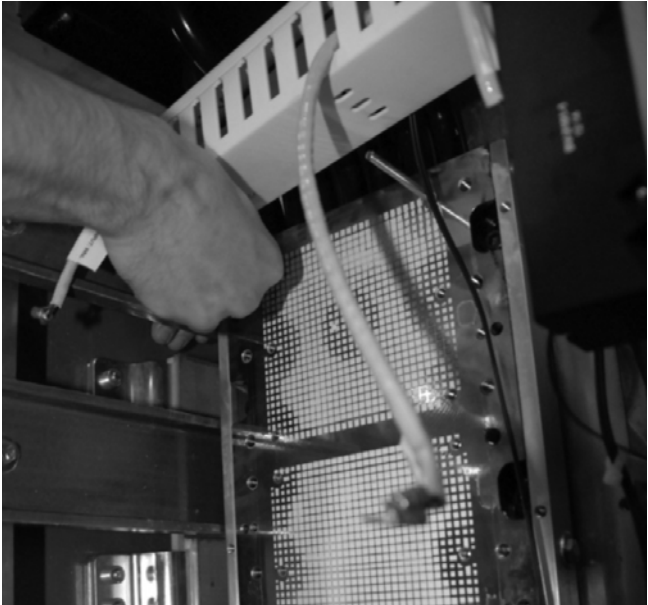
Figure 31. Install tapered pins for aligning power pole
