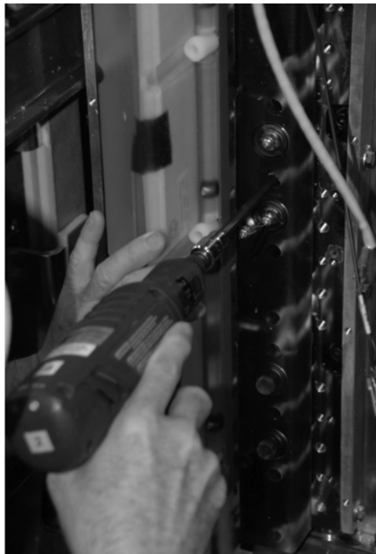
Figure 33. Secure hardware to power pole (wait 30 minutes and torque appropriately)
