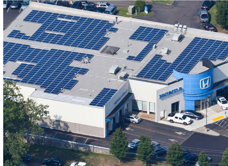
The solar roof at Brandfon Honda in Brandford, Conn. is one of the methods used by the dealership to be electric grid neutral.
