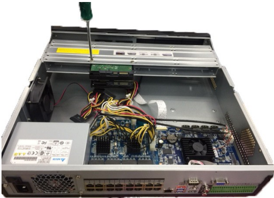
Figure 15-15 Placing the HDD
