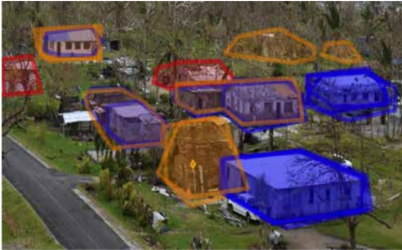
Oblique imagery taken from a drone used in damage assessment
