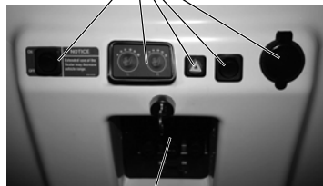
Electrical Access Panel (Fuses/Main Disconnect Switch)
