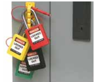
Step 5: Low-profile lockouts allow panel doors to be closed on most breaker panels.
