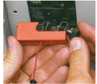
Step 2: Attach the lockout device to the breaker and snap into locked position.
