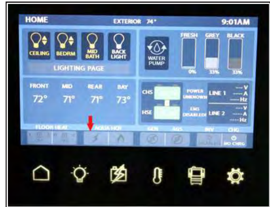
Figure 13-14: Hydraulic heating system
