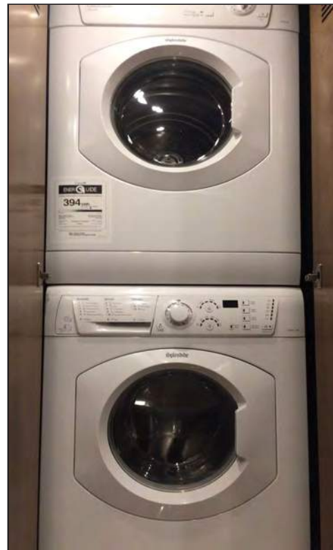
Figure 5-7: Stacked washer and dryer
