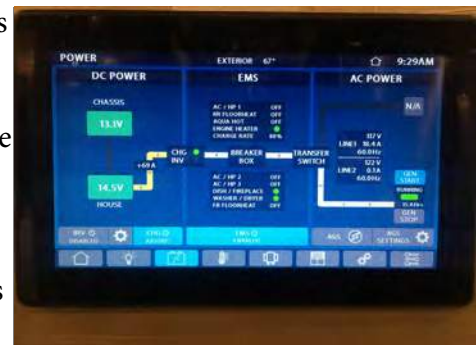
Figure 9-14: Energy management system
