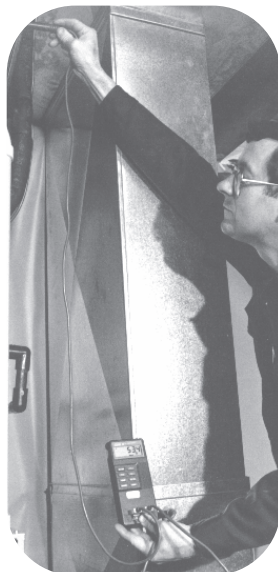
FIGURE 48 TEMPERATURE RISE MEASUREMENT
