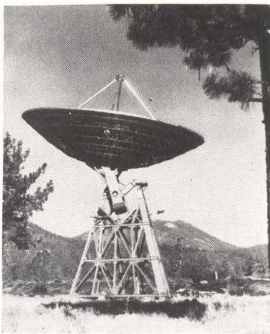
Single 70-ton counterweight balances 85-foot telescope in any position
