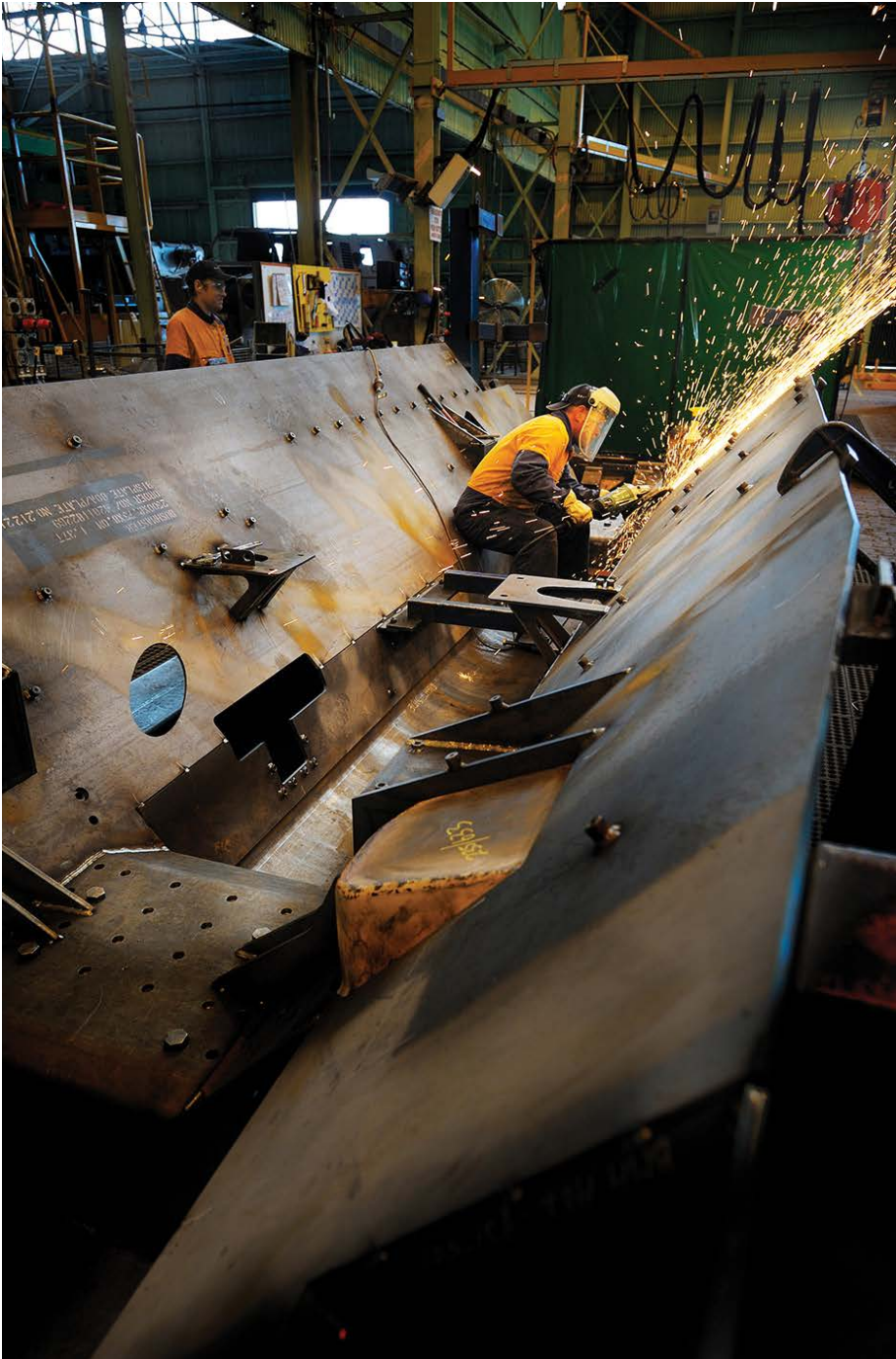
Building the Bushmaster from the V-shaped hull up at the Thales plant in Bendigo, Victoria. Photo courtesy of Thales.
