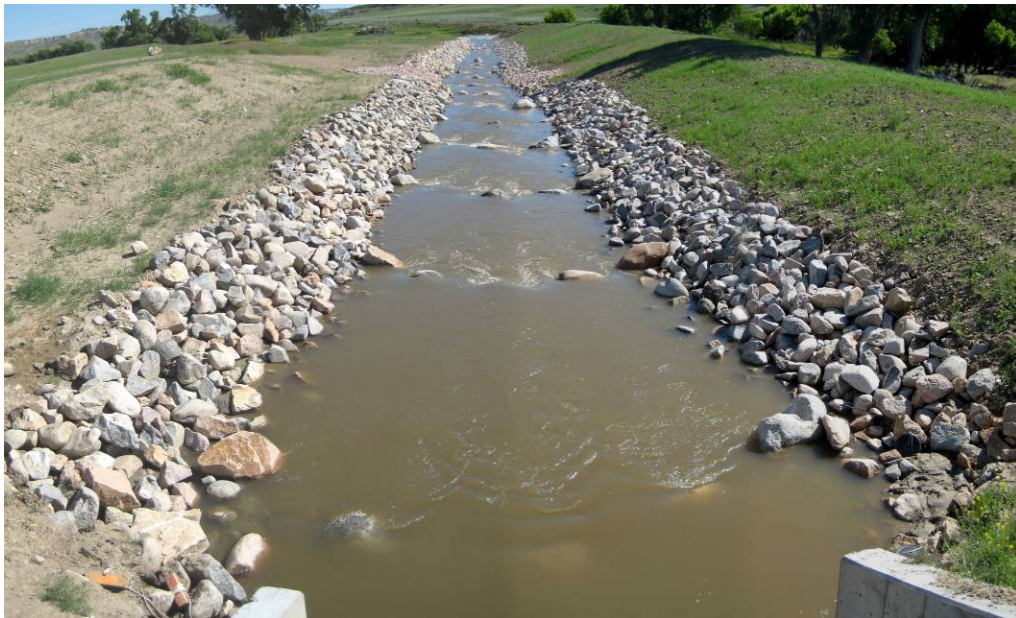
Fish by-pass channel (stepped)
