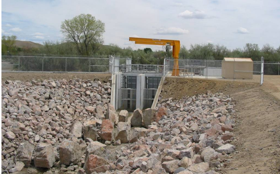
Fish passage structure with sorting facility (under construction)
