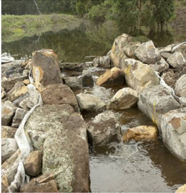
Low flow stepped boulder fish passage structure
