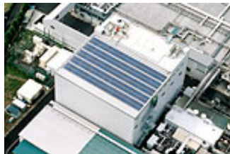
■ Kagoshima Hayato Plant (40 kW) (introduced in FY2006)
