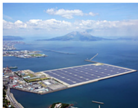
Kagoshima Nanatsujima Mega Solar Power Plant
