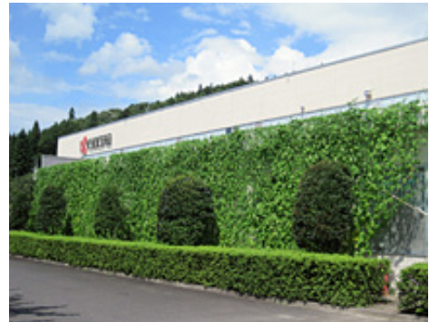
Green Curtains (Fukushima Tanagura Plant)
