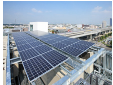
Roof of the Advanced Chemical Technology Center
