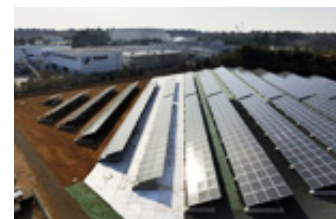
■ Chiba Sakura Plant (493 kW) (introduced in FY1985 and expanded in FY2014)
