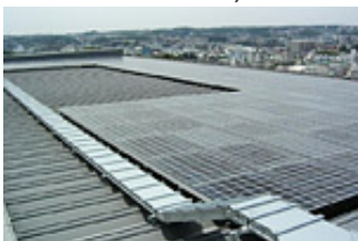
■ Yokohama Office (58 kW) (introduced in FY2012)
