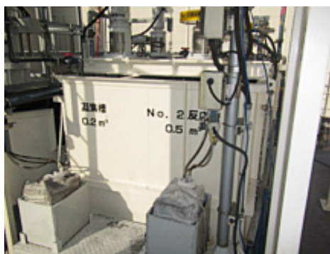
Cutting effluent treatment equipment
