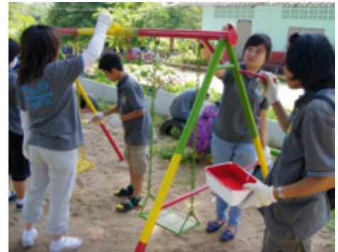
Volunteers building a playground at Ban Huai Hom School
